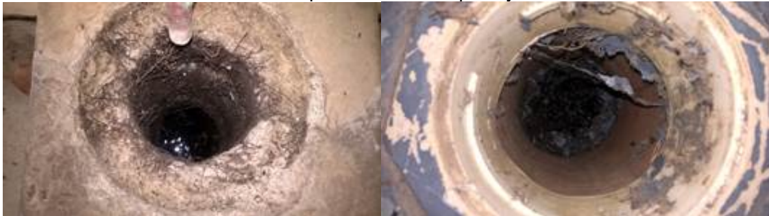
Tree roots penetrating waste internal pipes
