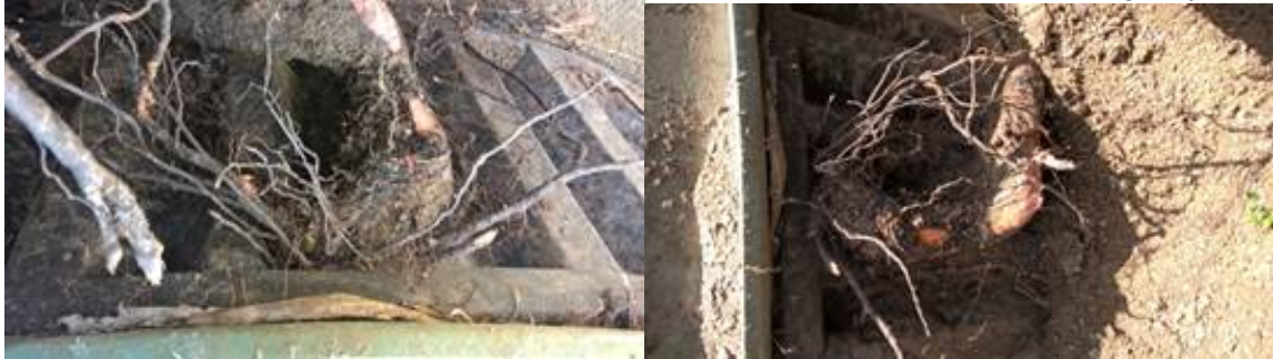
Tree root penetration of septic system tank.
