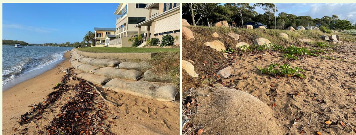
Figure 24. Existing conditions at Lilley's Beach entrance.
