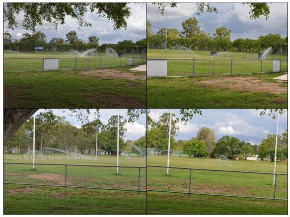
**Figure 8.6:** Irrigation station on AFL Oval operating as a single station (upper left) and in conjunction with another station (upper right). Further examples of low operating pressures in the lower images.
