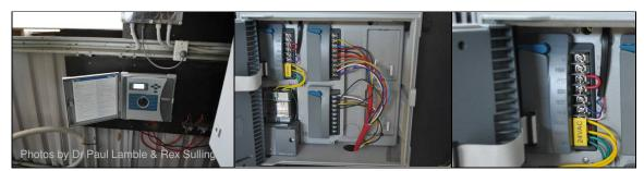
Figure 8.5: Irrigation controller (left) and control cabling (centre), with remote controller connection (right).
