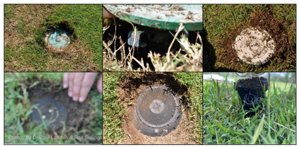
**Figure 8.7:** A sampling of the many different types of sprinkler present at the BITS Golf Course greens – Rain Spray, Rapid Rain, Rain Bird Eagle 700, Perrot and Hunter I-25.
