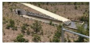
Figure 23 – Example of Scour Protection
