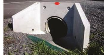
Figure 18 - Example of Headwall
