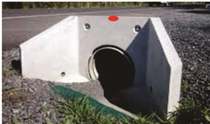
Figure 18 - Example of Headwall
