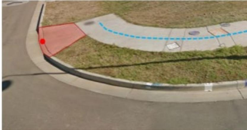
Figure 30 – Example of Kerb Ramp Asset
