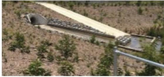
Figure 23 – Example of Scour Protection
