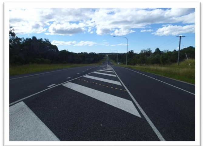
Figure 9 - Example of 1 Rural (1R) Sealed Road Service Level
