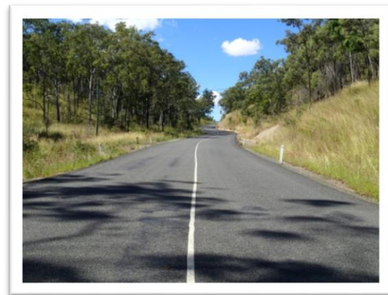
Figure 14 - Example of 3 Rural (3R) Sealed Road Service Level
