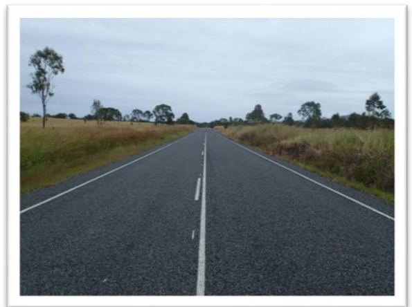
Figure 11 - Example of 2 Rural (2R) Sealed Road Service Level
