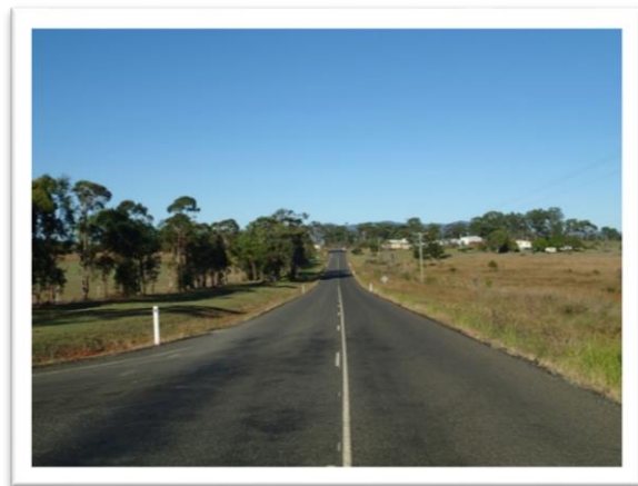
Figure 15- Example of 4 Rural (4R) Sealed Road Service Level
