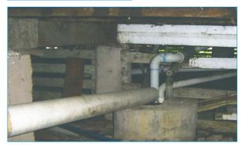
Illegal plumbing. The pipe from the right channels stormwater into the ORG.
