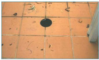
Paving that incorrectly channels water into the sewer system.
