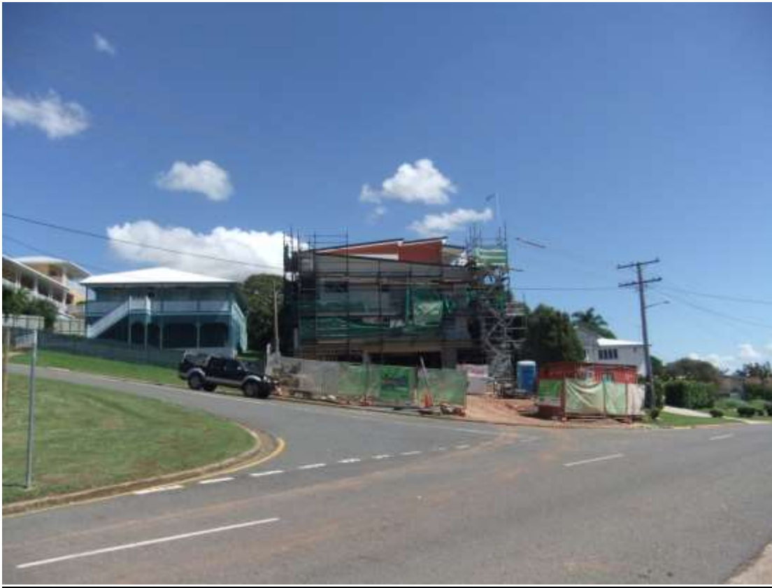
Construction Works - Corner Scenery & Bayne Street
