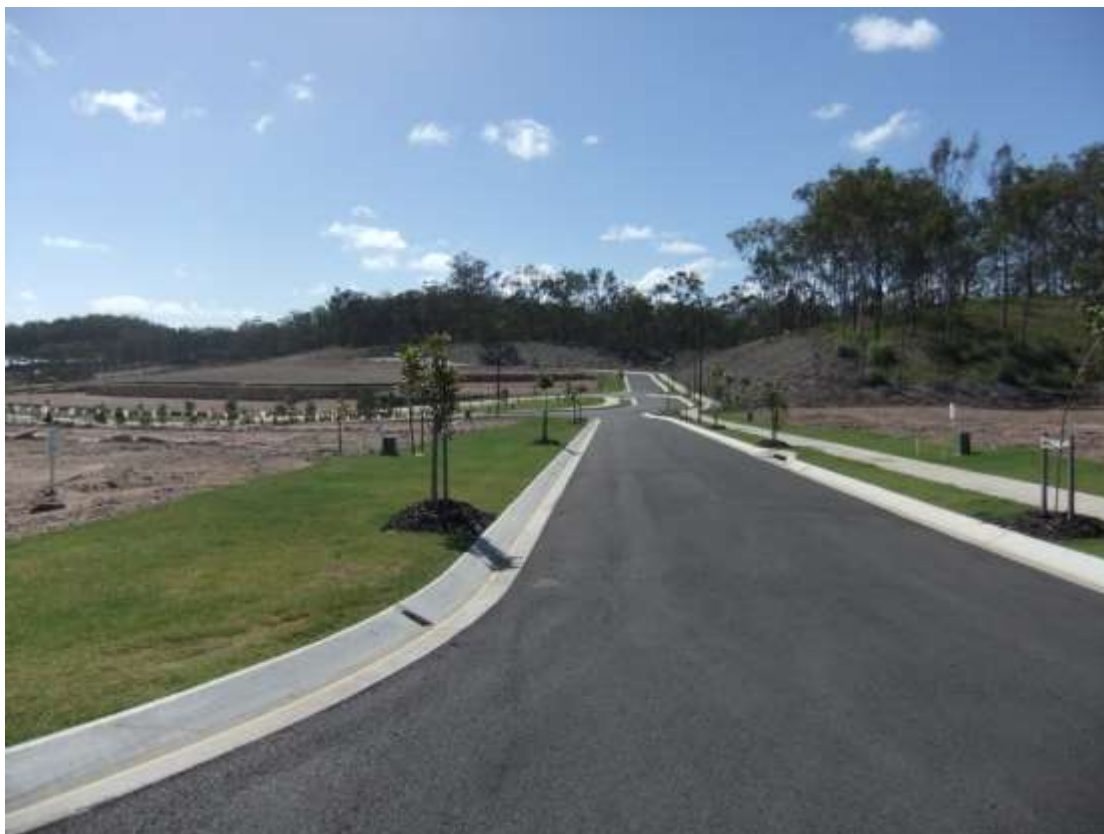
Construction Works - Stage 4B
