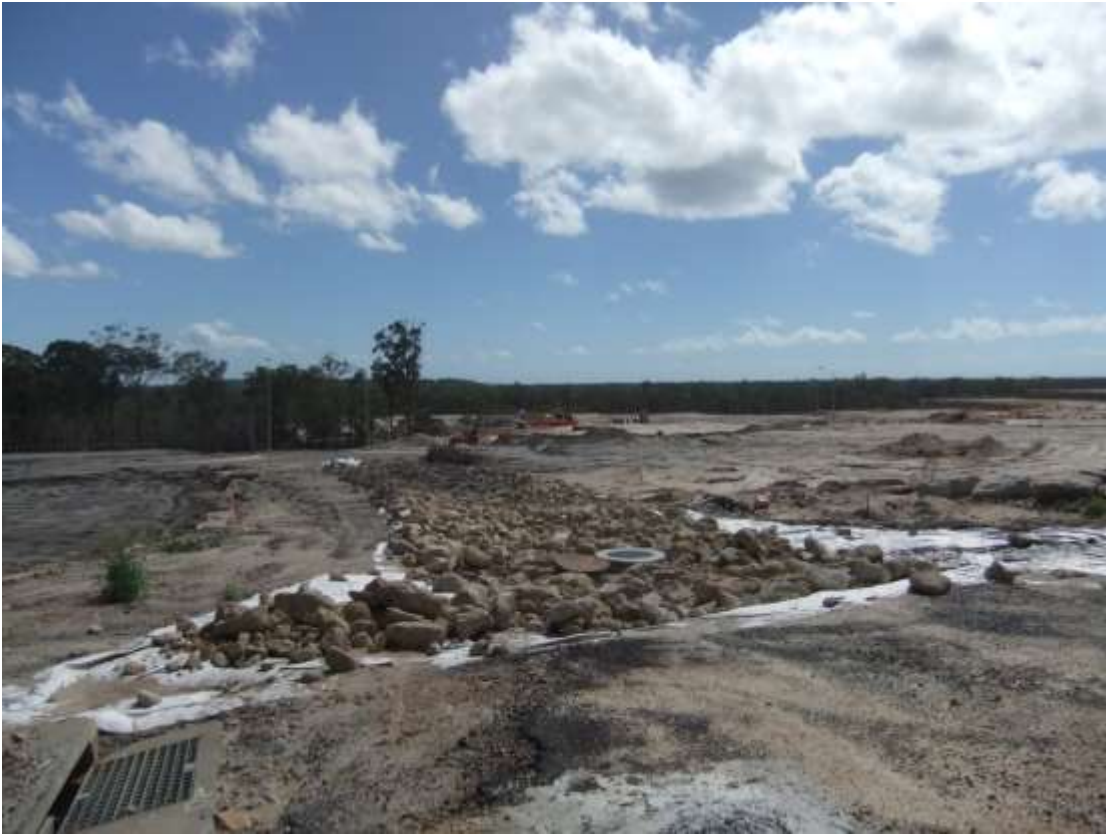
Construction Works - Spinnaker Drive
