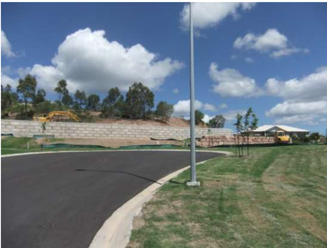
Construction Works - Dorinda Close
