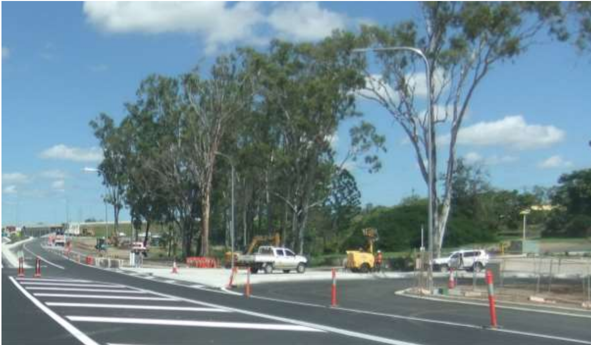
Construction Works - Dawson Highway Entrance
