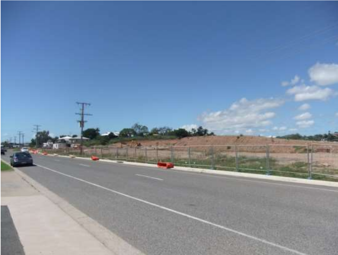
Construction Works - Chapple Street
