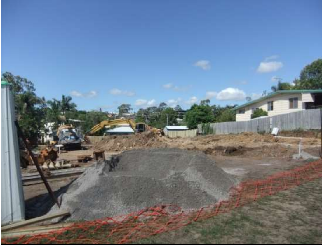
Construction Works - Crest Avenue
