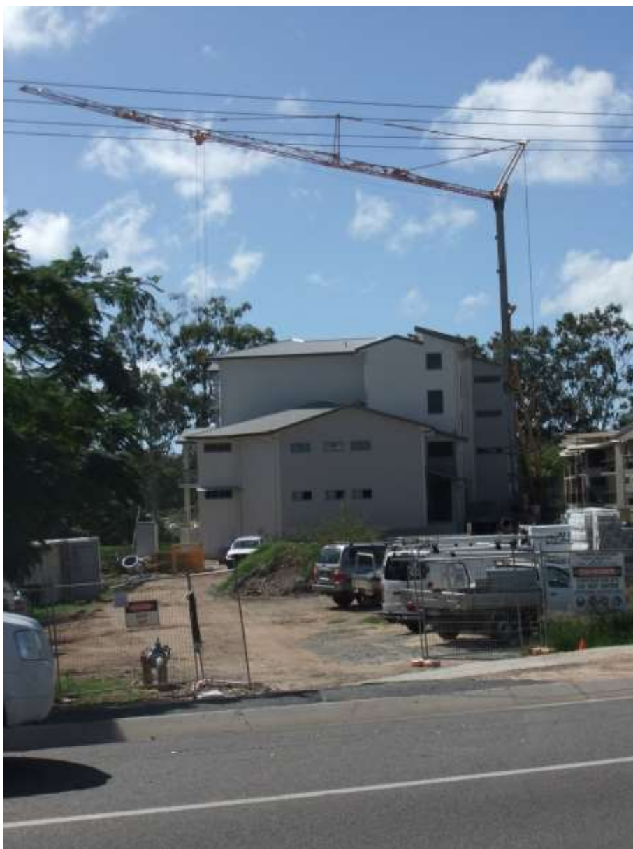
Construction Works - Wyndham Avenue
