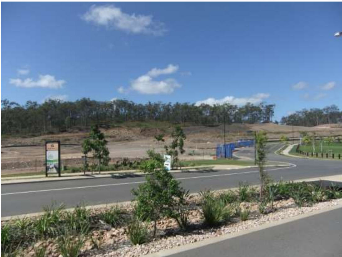
Construction Works - Stage 4A
