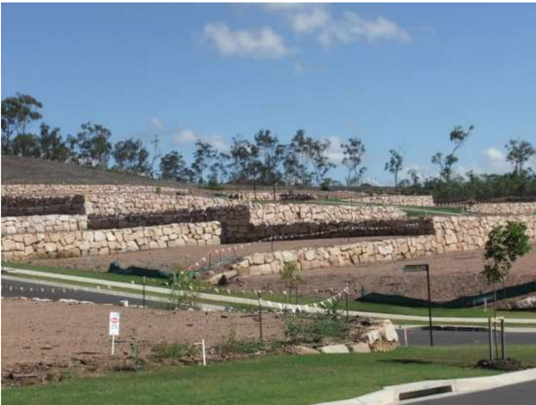
Construction Works - Stage 4B
