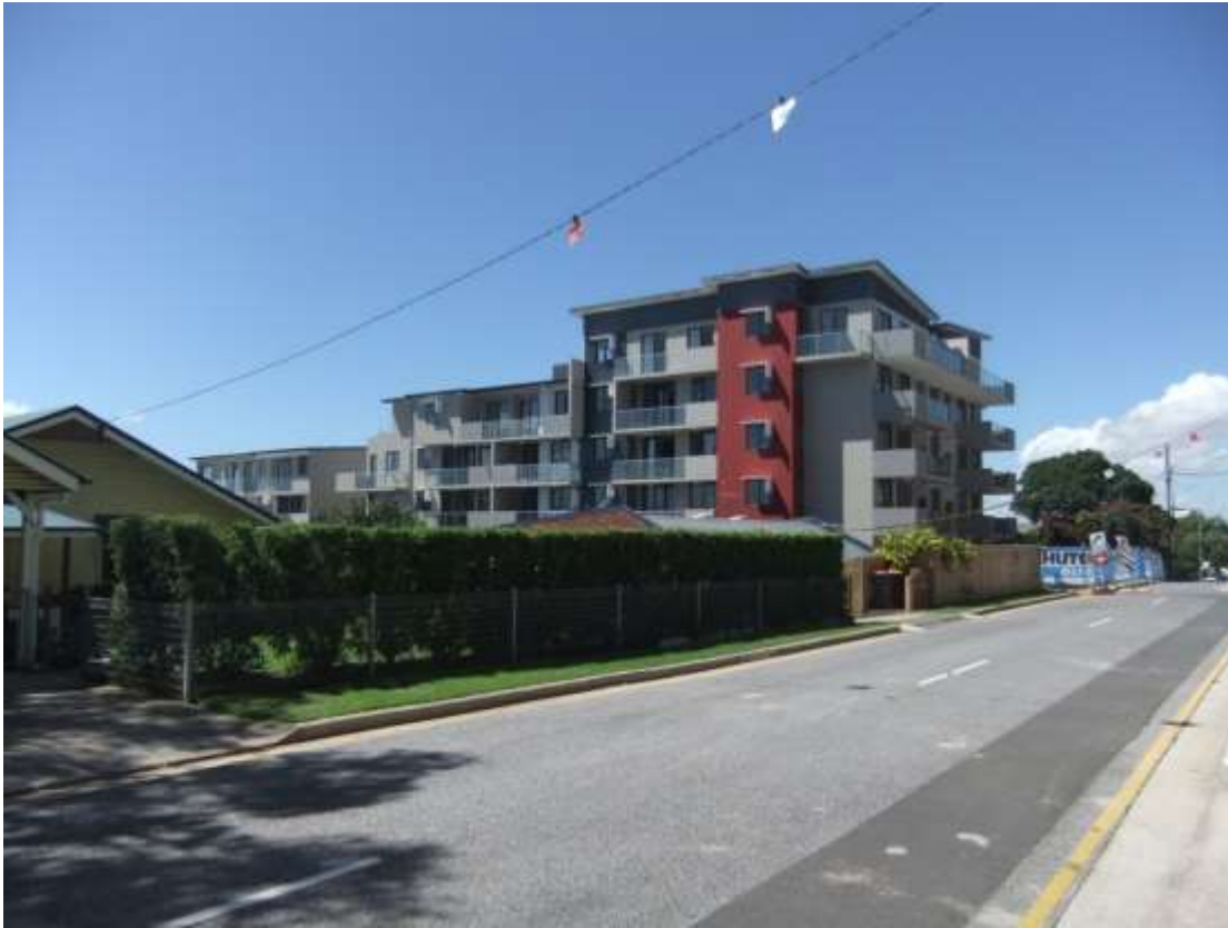
Construction Works - Oaka Lane
