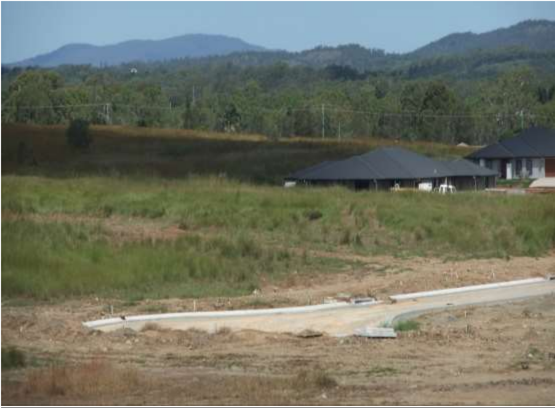
Construction Works - Stage 5
