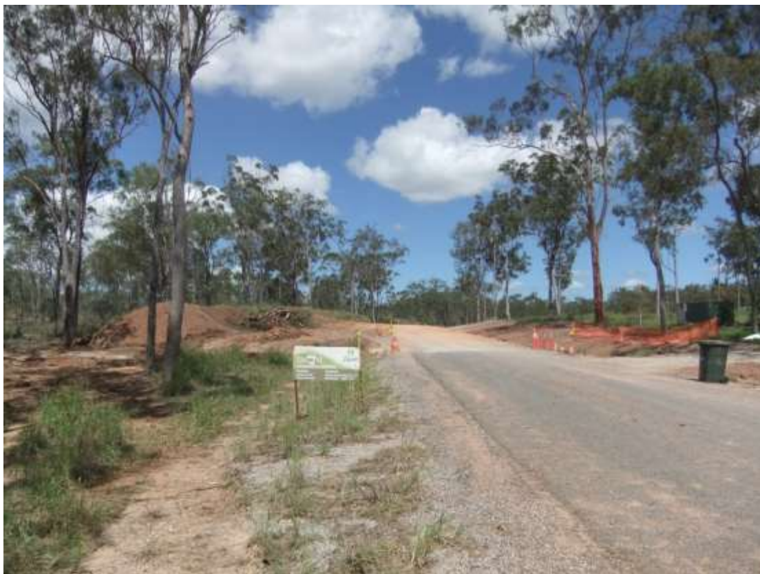
Construction Works - Brendonna Road
