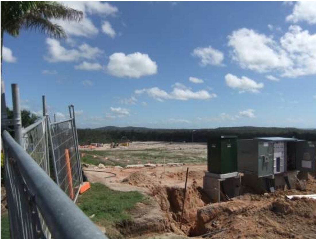
Construction Works - Broadacres Drive
