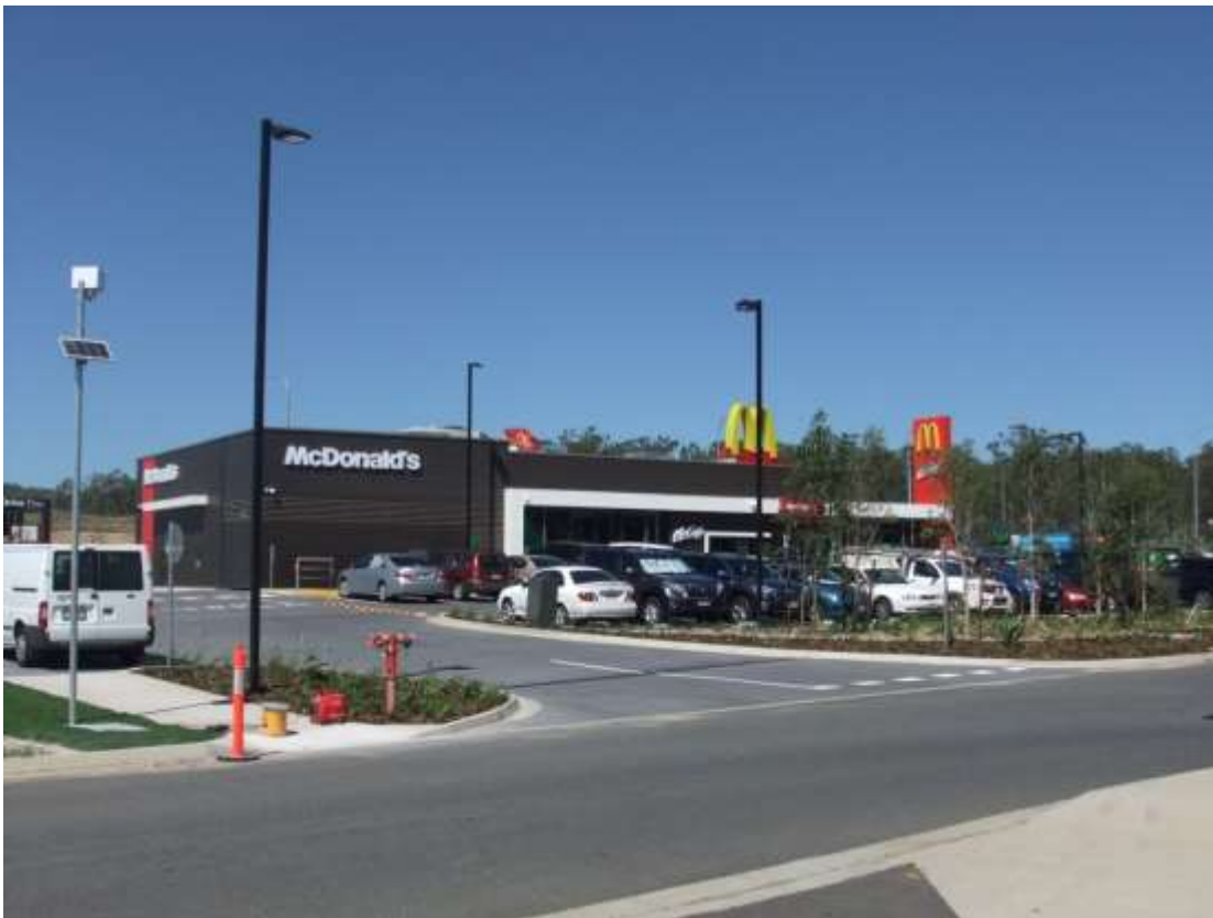
Construction Works - Corner Kirkwood Road & Dixon Drive
