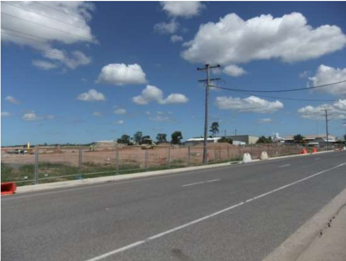
Construction Works - Chapple Street
