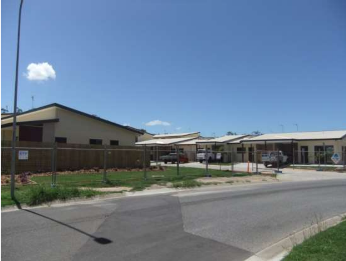
Construction Works - Pioneer Drive
