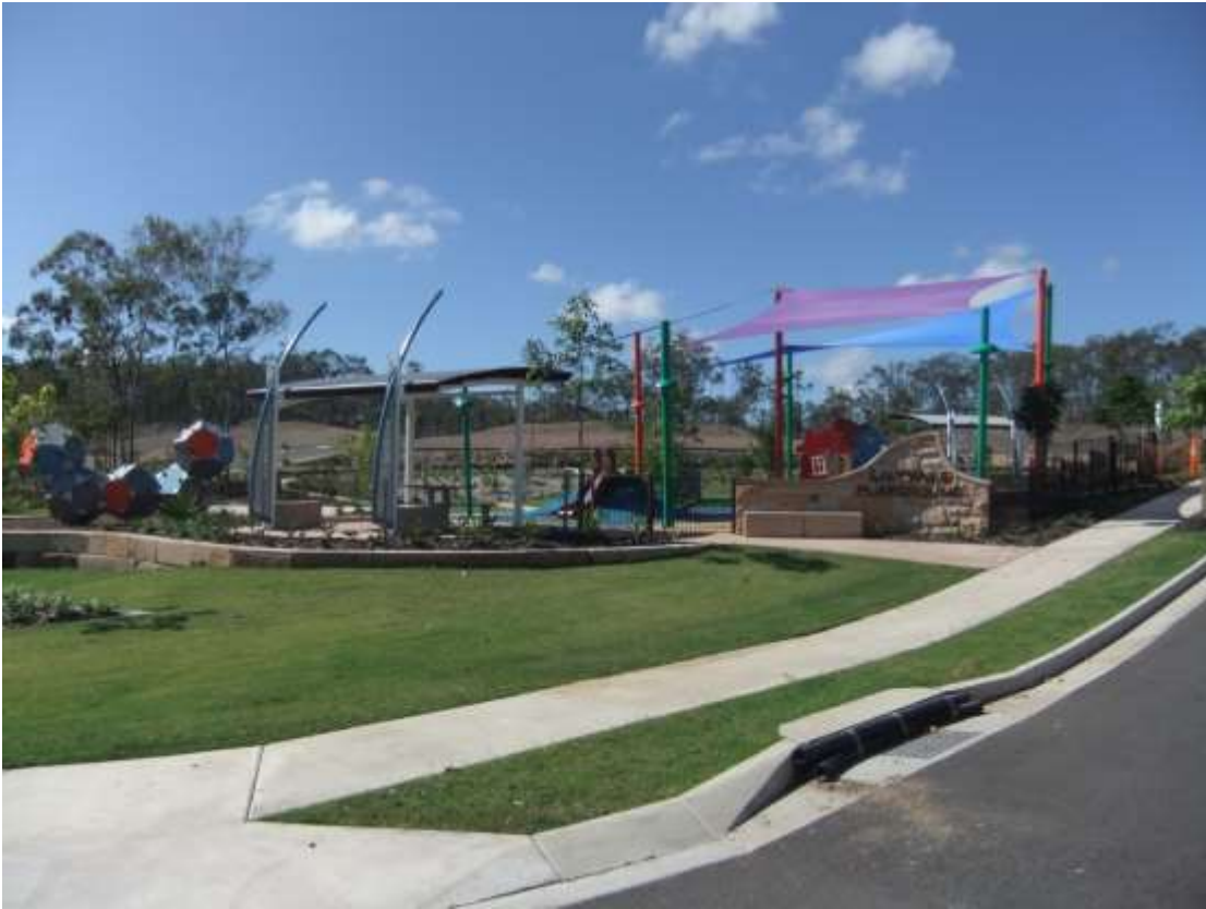
Construction Works - Stage 4B Park
