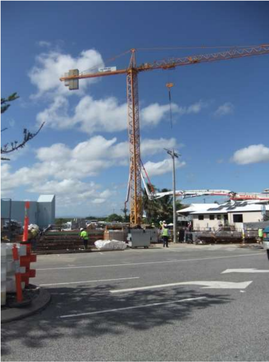
Construction Works - Pacific Avenue
