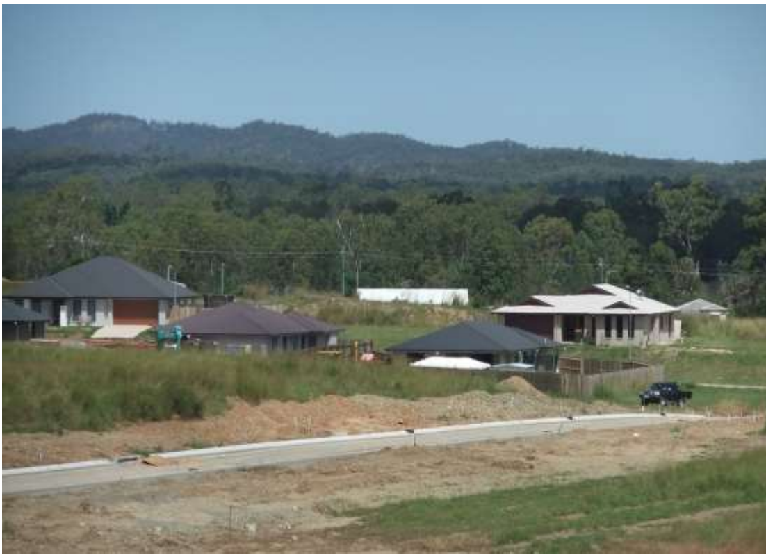
Construction Works - Stage 5
