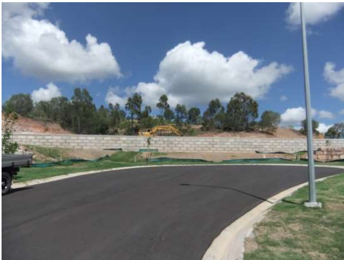
Construction Works - Dorinda Close
