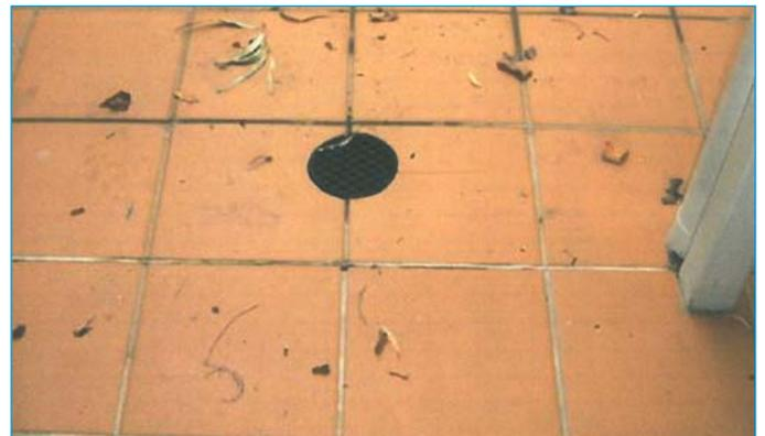
Paving that incorrectly channels water into the sewer system.
